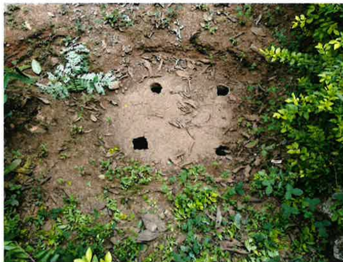
Rainwater Harvesting Pit
